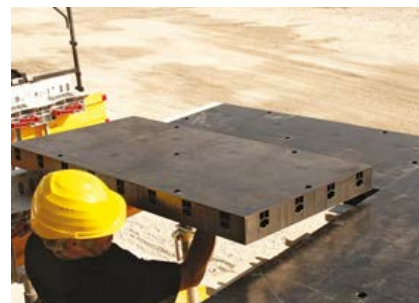
③ POSA PANNELLI GEOPANEL
