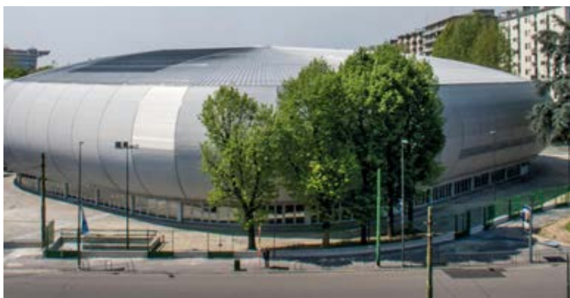
DRAINPANEL Allianz Cloud Sport Hall MILANO, ITALIA
