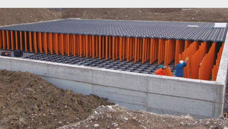
SYSTEM MADE OF RECYCLED PLASTIC MATERIAL USED TO CREATE CONCRETE TANKS FOR RAINWATER HARVESTING OR INFILTRATION. SYSTEM ADJUSTABLE TO HEIGHT AND DIMENSIONS OF THE TANKS, AS PER DESIGN REQUIREMENTS.
