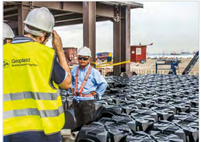
On-site assistance for Modulo formwork
