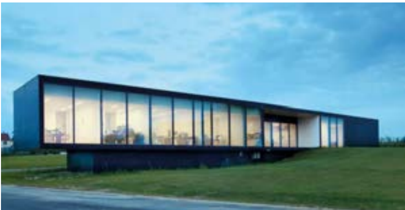
DRENING Marchesini Group HQ PARIS, FRANCE
