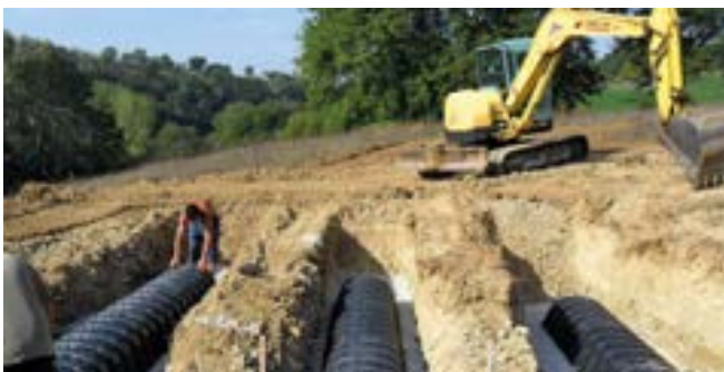
③ INSTALLATION OF DRENING Install the Draining chambers.
