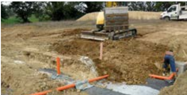
⑤ LAYING OF GETOTEXTILE Lay geotextile over the whole surface.
