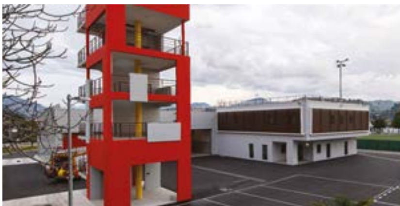
ELEVATOR TANK Firefighting center SAINT-LAURENT-DU-VAR, FRANCE
