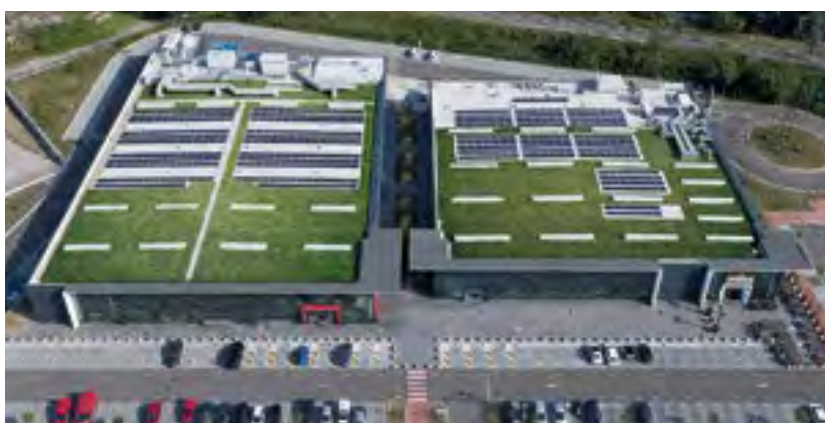
COMPLETA, 3200 m 2 SUPERMARKET BOLOGNA, ITALY
