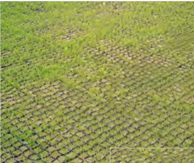
Green area with Runfloor 58 F03 For the transit and parking of vehicles.
