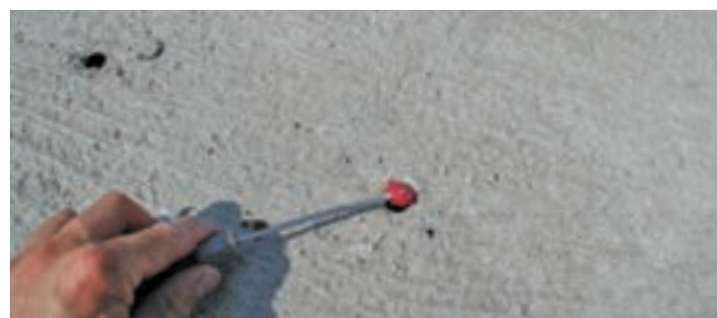
⑥ REMOVING THE CAPS Remove the nozzle end caps to allow the air to flow into the system.
