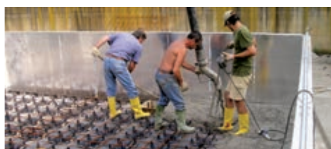
④ POURING Concrete pouring as per design spec.
