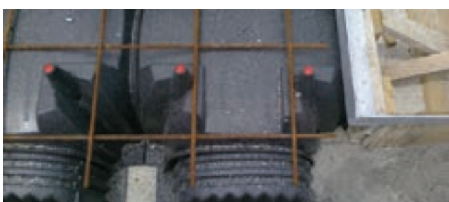
③ STEEL MESH INSTALLATION Install the reinforcements as per design spec.
