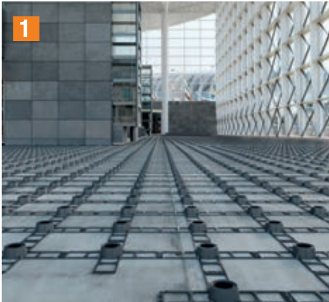
1 The Matrix base-grid facilitates installation by clearly indicating the available routing for utilities.
