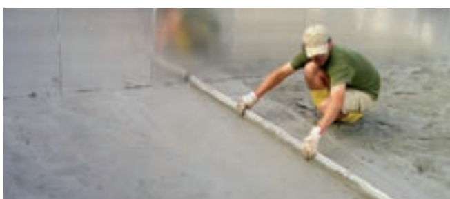
⑤ CONCRETE LEVELLING Level the concrete in order to obtain a uniform slab.
