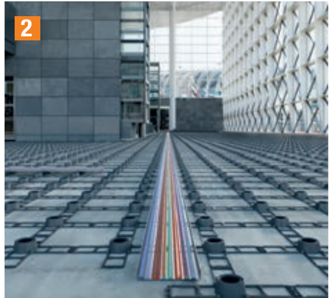
2 Lay cable ducts, electrical tubes and pipes as per design requirements.
