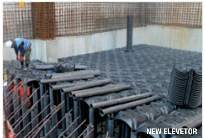
New Elevator Formwork
