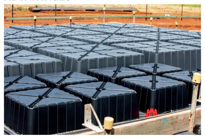
The spacer is specifically designed to allow sequential laying of the pods alternated with the spacers. Geopod is made of 100% recycled PP compound, in line with Geoplast focus on Green Building and Sustainability. The product offers great logistic advantages in comparison with the traditional waffle pods in EPS, with about 95 Sq.Mt. of ground slab that can be shipped in one pallet H180.
