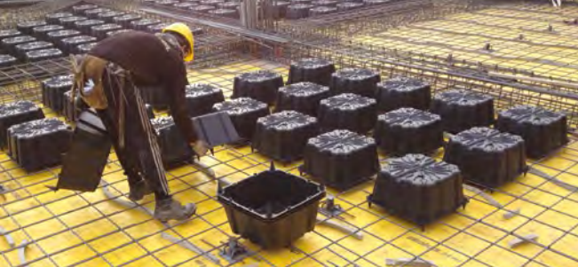
③ LAYING NEW NAUTILUS
