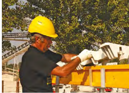
② LAYING TRAVELLETS H
