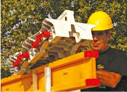
① LAYING TRAVELLETS Y + C
