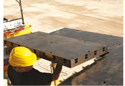
③ LAYING GEOPANEL PANELS
