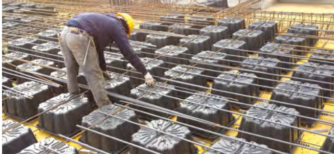
④ COMPLETION OF LAYING ARMOUR
