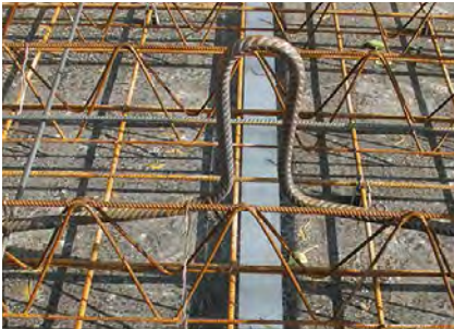
④ LAYING ARMOUR
