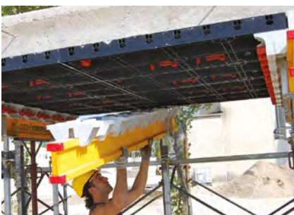
⑥ H JOIST REMOVAL
