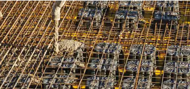
⑤ FIRST PHASE CASTING
