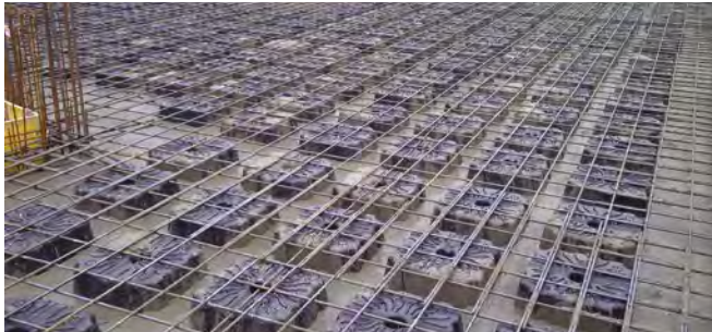
⑥ WAITING BETWEEN FIRST AND SECOND JET PHASE
