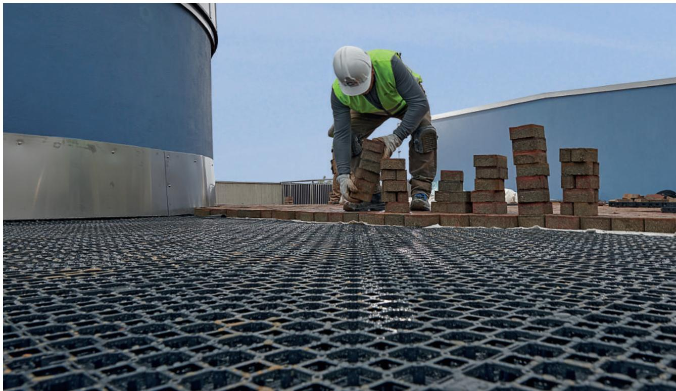
Geocell is a high-strength grid made of regenerated polypropylene for wide-area water drainage underneath paved areas.
