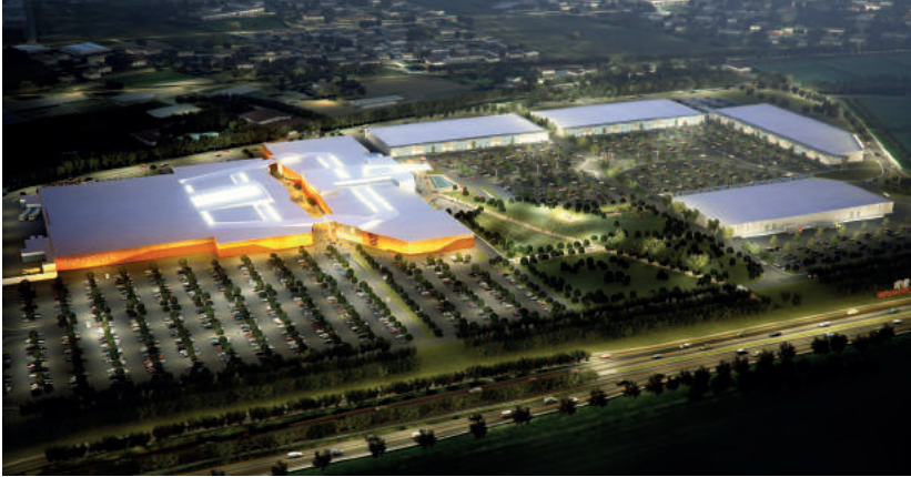
ELEVATOR TANK MondoJuve shopping mall TORINO, ITALY
