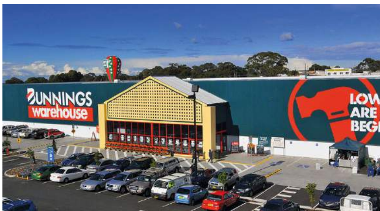
Bunnings Warehouse SYDNEY, AUSTRALIA
