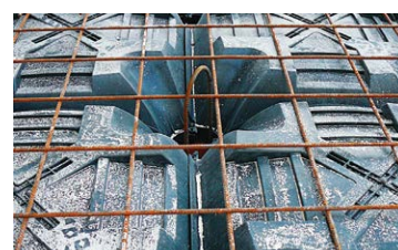
Reinforcement of the pillar with steel forks
