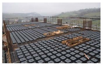
Figure 59 - preparation of cavities before casting
