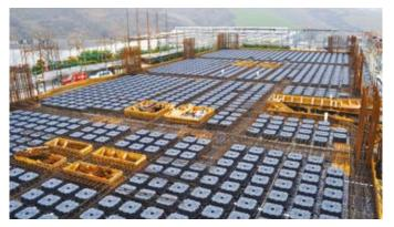
Figura 1 - lightened slab with New Nautilus Evo of Geoplast.
