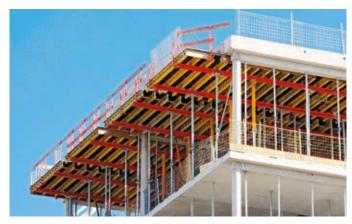
Figure 39 - formwork of cast-in-situ slab with traditional wooden formwork and plywood panels
