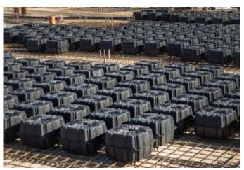
Figura 3 - layout of lightening New Nautilus Evo double
