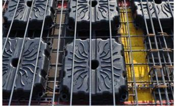
Figure 49 - placing of the upper reinforcement bars
