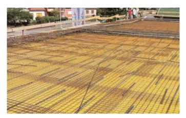
Figure 41 - laying of the lower reinforcement mesh
