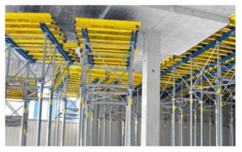
Figure 40 - formwork of cast-in-situ slab with modular wooden formworks
