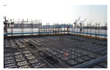
Figure 50 - laying of the upper reinforcement bars
