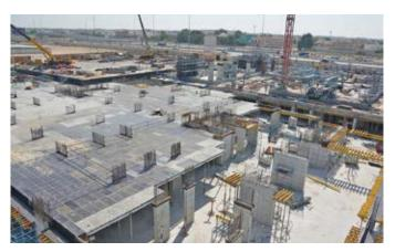
Figure 38 - formwork of cast-in-situ slab with modular metal formworks
