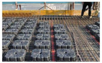
Figure 46 - layout of lightening
