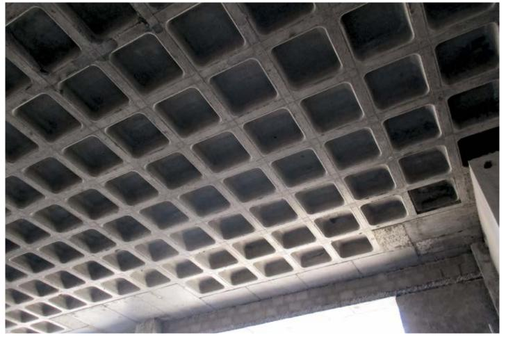
Figure 2 - example of reticular slab
