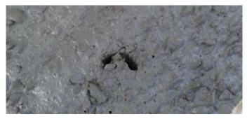
Figure 57 - the impression in the concrete indicates the right time to resume the casting
