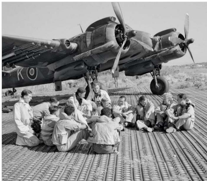
During the Second World War the allies developed a system of perforated and modular steel grids, called “Marston Mats”, which stretched on the ground and united to others were used for the rapid preparation of airports and roads. The Italians called them “perforated metal grids”, neologism derived from the English term “grill” that means grid.
