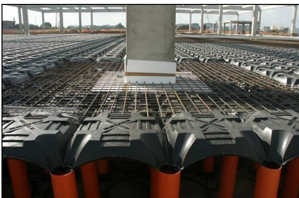
Fig. 3 Slab thickening around the columns
