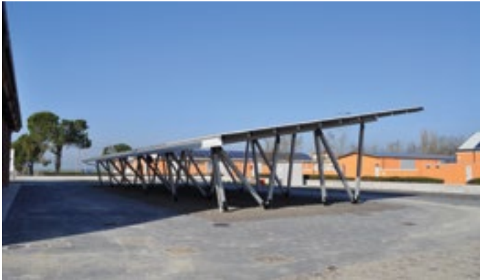
Figure 12 - Completion with parking finish
