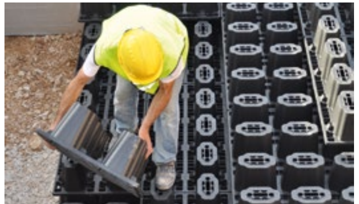
Figure 17 - Installation of Drainpanel
