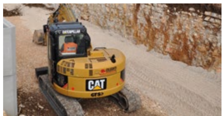
Figure 11 - Drainpanel system covering and re-filling phase
