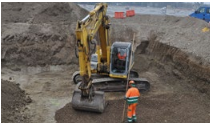
Figure 16 - Excavation phase and background preparation
