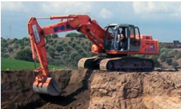
Figure 7 - Excavation and background preparation
