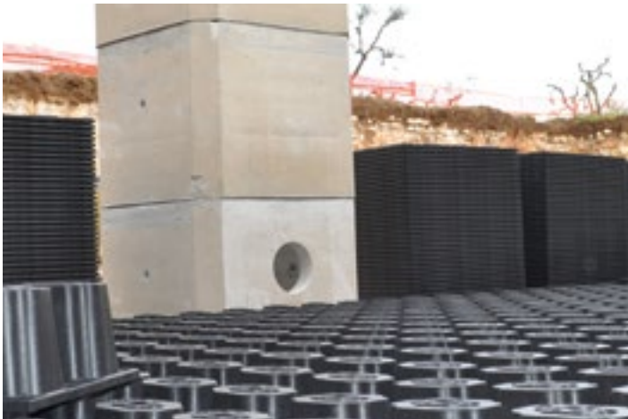
Figure 21 - Point of access to the inspection system
