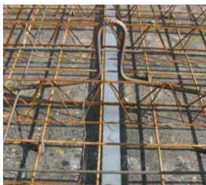
④ INSTALLATION RENFORCEMENT
