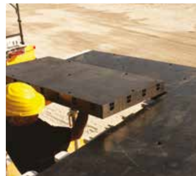
③ INSTALLATION PANNEAUX GEOPANEL
