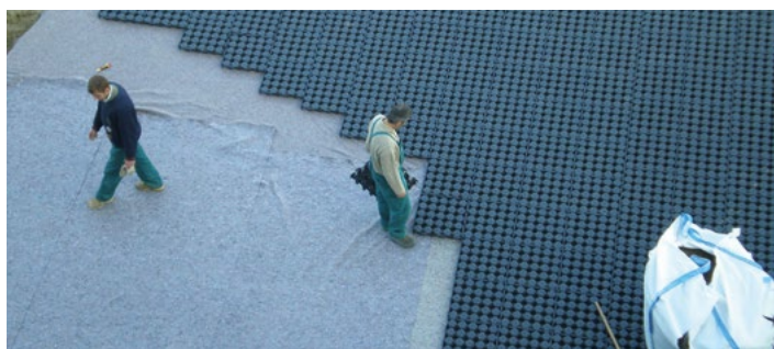
Figura 11 - Posa in opera Drainroof
