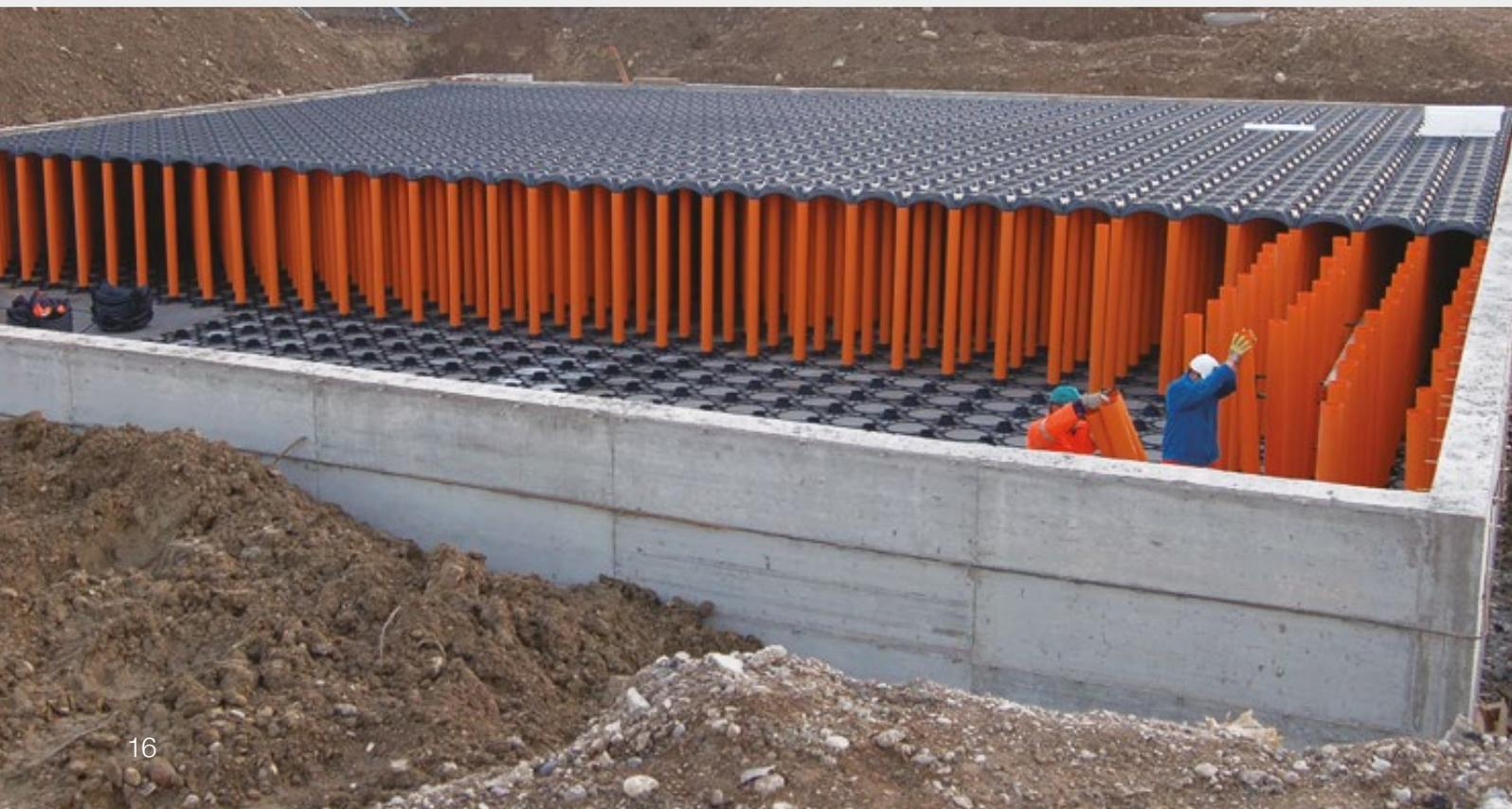
**SYSTEM MADE OF RECYCLED PLASTIC MATERIAL USED TO CREATE CONCRETE TANKS FOR RAINWATER HARVESTING OR INFILTRATION. SYSTEM ADJUSTABLE TO HEIGHT AND DIMENSIONS OF THE TANKS, AS PER DESIGN REQUIREMENTS.**
